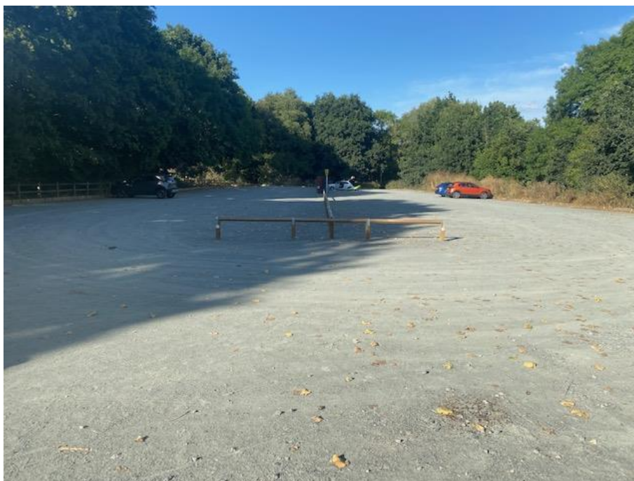
Teston Bridge overflow car park following resurfacing
